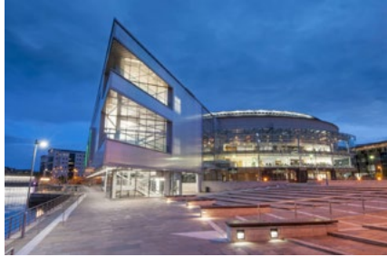
Belfast International Conference Centre (Syncimaging, Courtesy of ICC Belfast)
